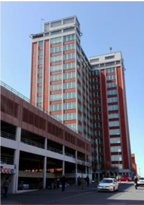
Figure 1. Former factory premises – Building No. 21
