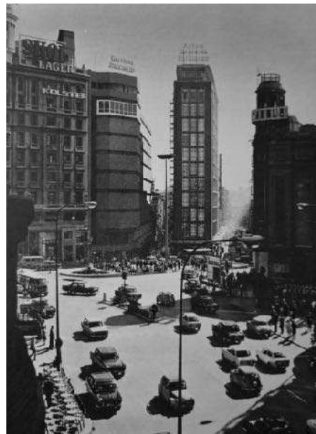
Figure 20. The newly developed Plaza del Callao. In the background, Galerías Preciados (3rd ed., 1971)
