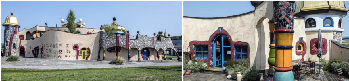
Figure 1. Markethall. Main façade and terrace. 1998 to 2001. Switzerland.
