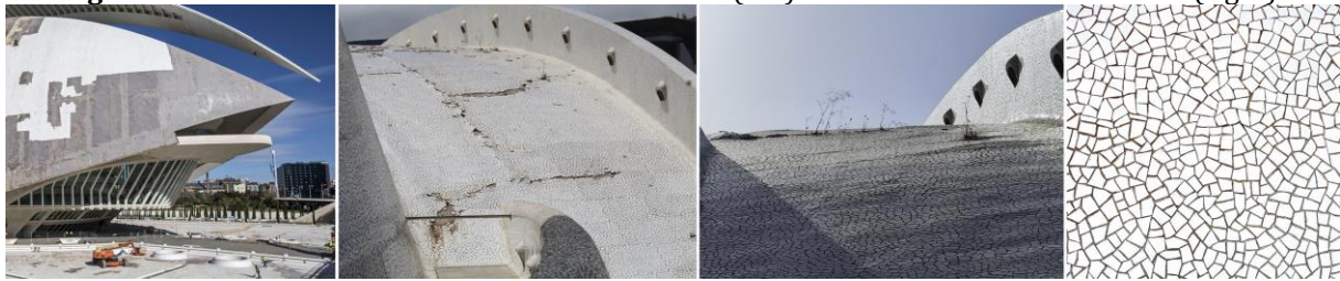
Figure 5. Facades of the Palau de les Arts Reina Sofía (left) and the Auditorio Adán Martín (right).
