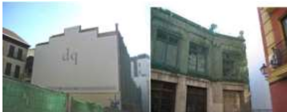
Image 3: The Serrería under construction 2000-2004
