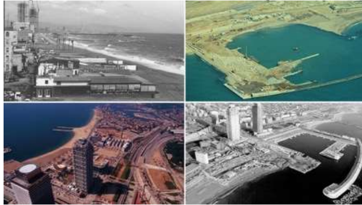
Image 5: Panoramic view of the works at the port of Barcelona
