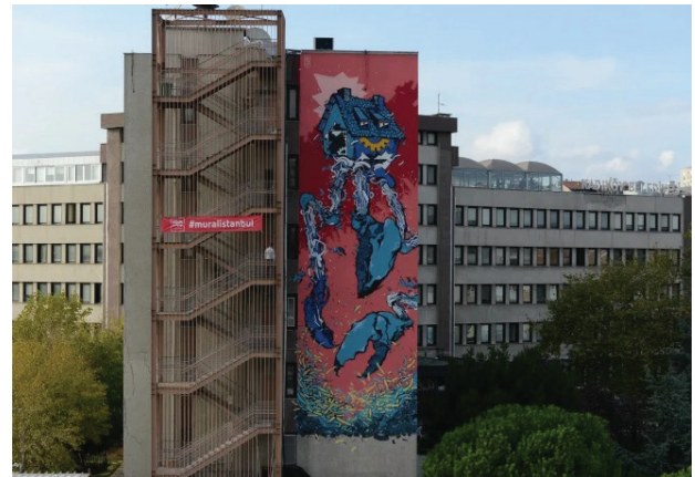
Figure 6. Work in Kadıköy Municipality building by Nuka, 2015 Author's photo
