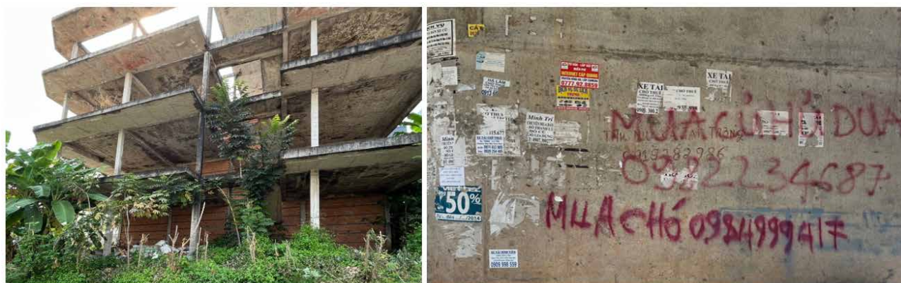
Figure 5: Abandoned construction, advertising stickers, and dirty painting on the walls
